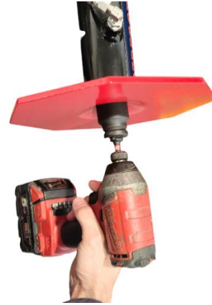
Step 2. Use an impact wrench to secure nut or bolt in place.
