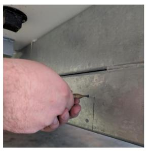
Use a punch to mark the center of the bracket hole, this will prevent the drill bit from walking.
