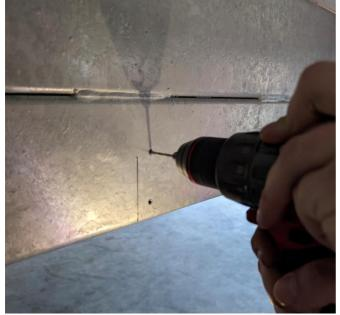
Before you start drilling, check which side of your chassis has the wiring loom. Make pilot holes with a 5mm drill bit, try not to go all the way through the chassis to avoid hitting any wires.
